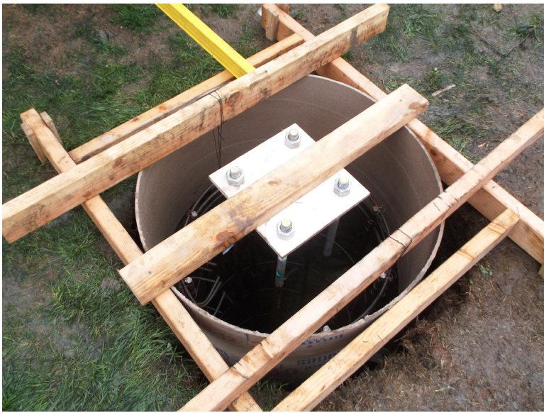
A template with the anchor bolts for the flagpoles is positioned.
